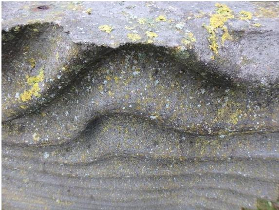
An Example for surface texturing of a concrete element
