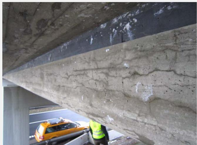
Photo: Severe surface ASR cracking in concrete bridge deck.
